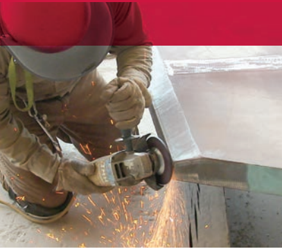
Grinding on a platform for weld preparation.
