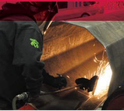
Weld removal with Tiger combo wheel.
